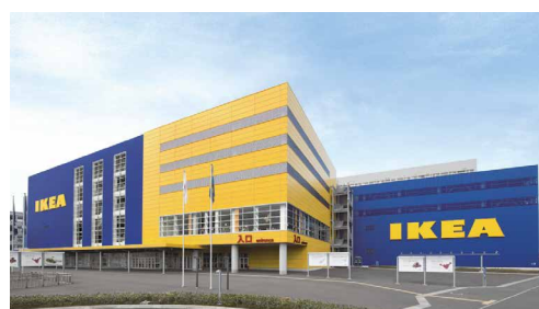
Exterior of store
